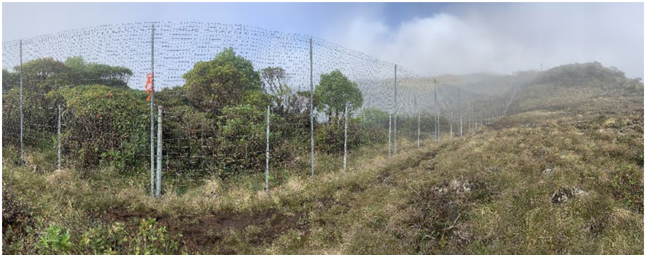
Fence project end point is flagged in triple orange.
