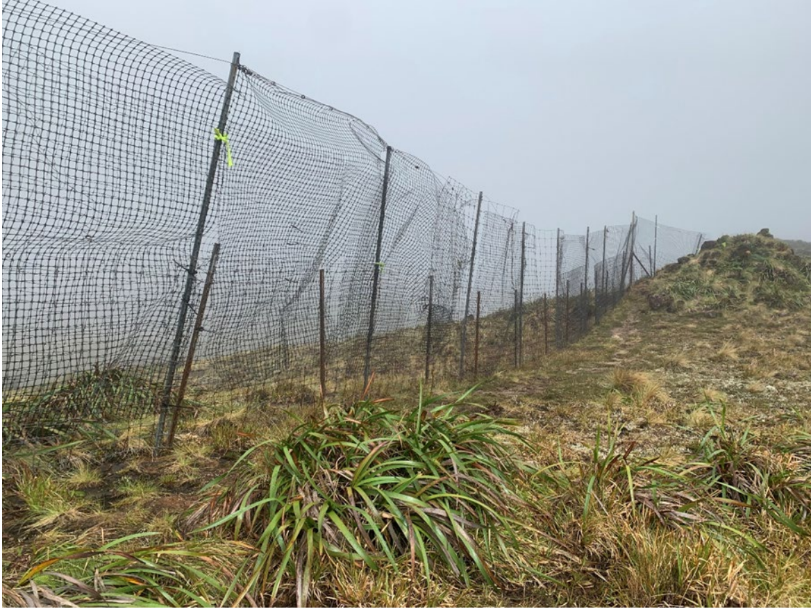
East Alaka'i Summit Fence currently contains a mix of materials. This image shows elk mesh, deer mesh, hog wire, and various ties.
