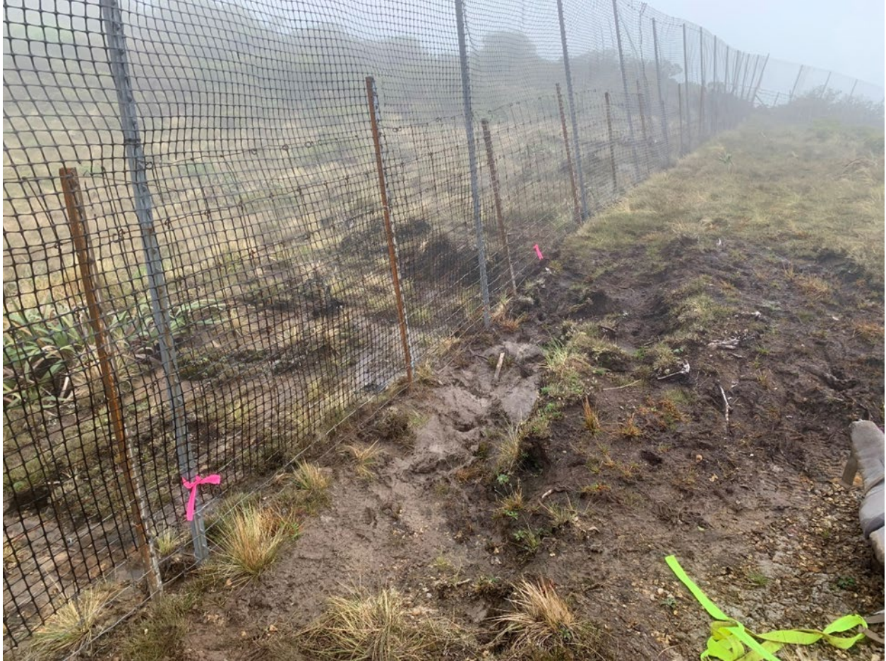
Pink flags indicate a muddy area where panel grate skirting is needed.
